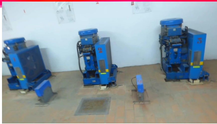
An Otis motor room with 3 Otis Europe (aka Edelma) motors and Otis mod logic controllers.
