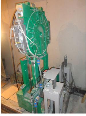
Here are some pics of an very small Kone Minispace Lift. It only got 3 Ropes and is based on the 4.th Generation Ecodisc. It got the NMX07 Hoisting machine and the LCECPU561. Minispace Lifts are never **MRL**
