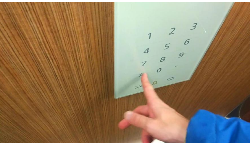
A very confusing Schindler 3300 with capacitive buttons and keypad floor selection. It was not clear when this lift wanted you to enter a floor and when you should enter an access code.
