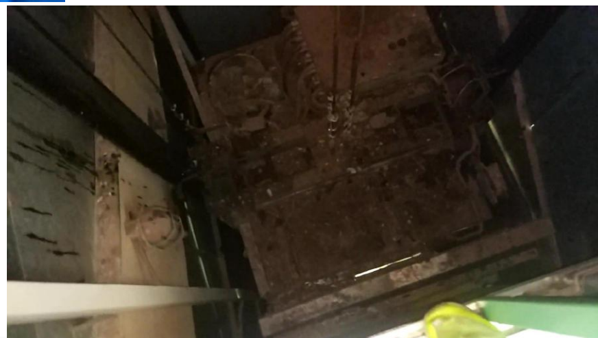
Some of the old lifts are badly maintained and do not have inspection controls
