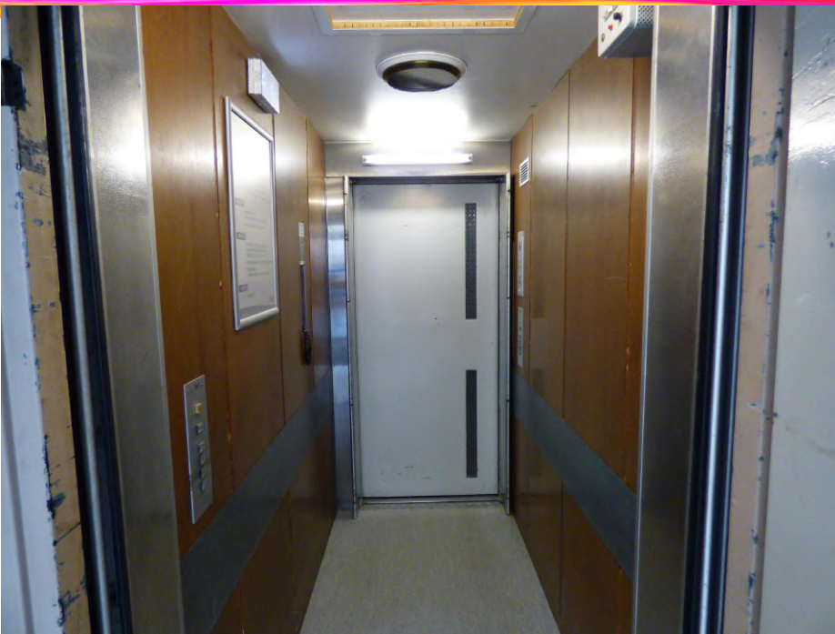
Left: A very interesting swing door lift in a hospital in Rennes.
