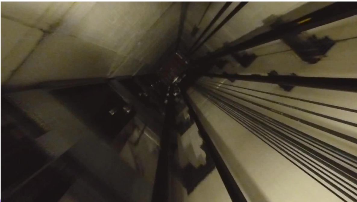
Lift shaft extended into the motor room space in a tower block and the lift was converted into a Thames Valley MRL with Zeta motor. It has side pulled 1:1 cabling and a side chassis
