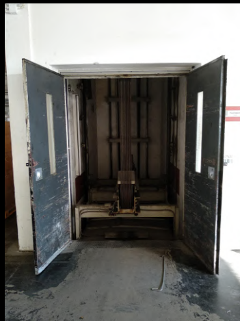
The BAAS Lift itself. No cartop controls, but a Long metal rod used to unlock doors
