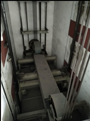
The BAAS Lift itself. No cartop controls, but a Long metal rod used to unlock doors
