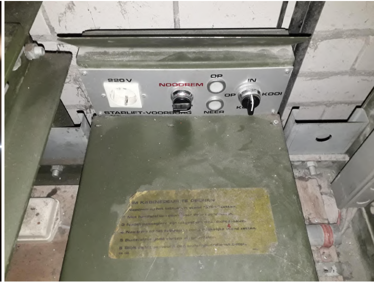
-90s Starlift and inspection panel
