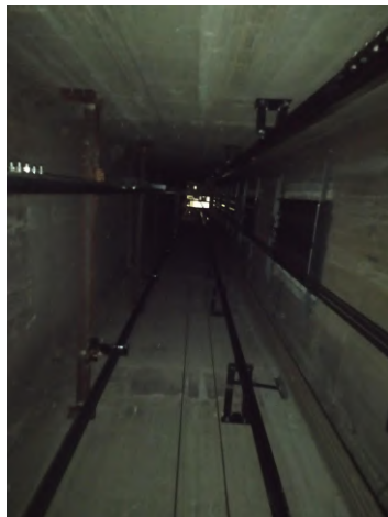
Brand new FUJI Lifts at Hospital Building. This lift has a speed of 1 m/s, very slow for a building of 10 floors,
