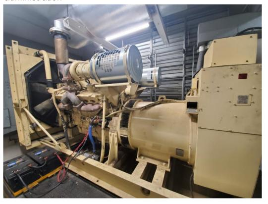
Here is a diesel generator for a datacenter. It's a six cylinder diesel engine with a giant alternator on it essentially. Since diesel is more sensitive to temperature, the fuel has to be heated. I've been told that checking the temperature of the fuel is part of the walk through that the datacenter operator has to do every so often. There are also two UPS' outside of the room this is in, they are there as standby as this thing takes a few moments to turn over and start supplying power.
