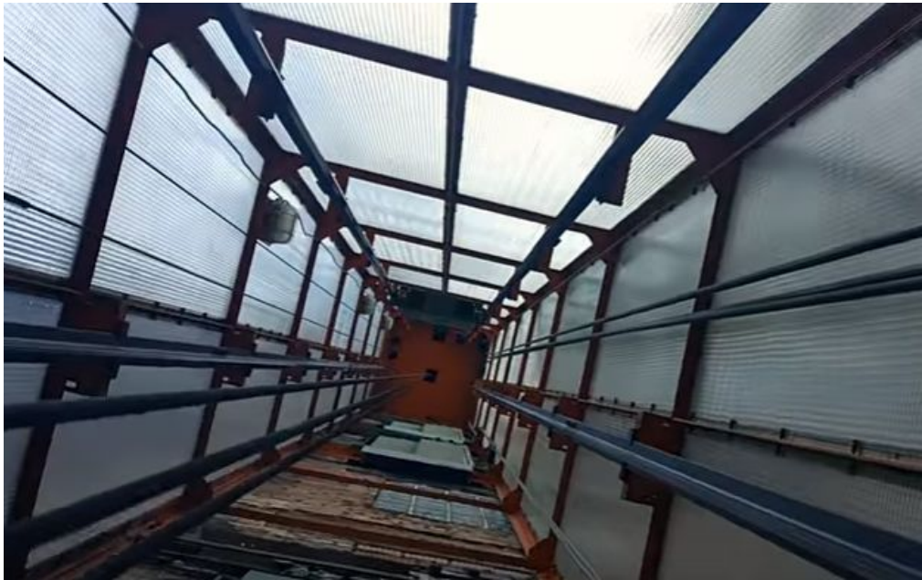
This Kleindienst Aufzuge was very interesting. The lift shaft is an extension to the building.
